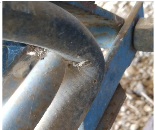
Figure 1. Crimps in hoses may lead to cracking.
