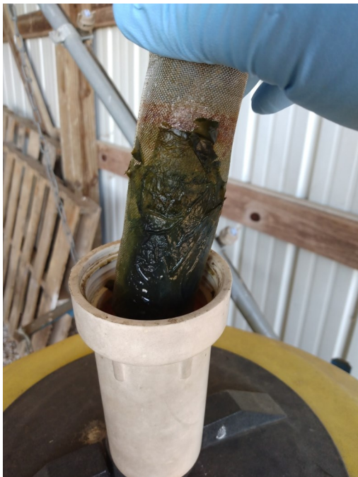
Figure 2. Check strainers regularly and clean or replace them as needed.
